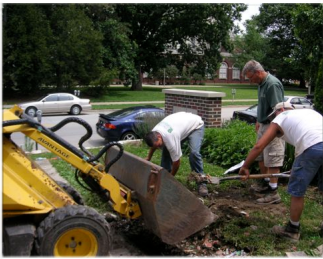
Demolition begins under Dan Swartz' watchful eye, our Landscape Architect
